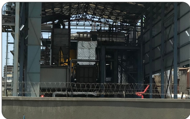
Benzo Chem Industries Pvt. Ltd. - Dahej, Gujarat Steam Boiler(IBR):- Capacity - 8 TPH, Fuel- Coal / FBC
