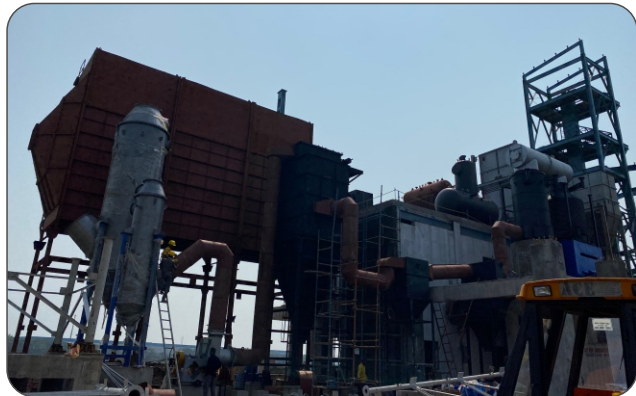
Privi - Bharuch, Gujarat Steam Boiler(IBR):- Capacity - 16 TPH, Fuel - Coal
