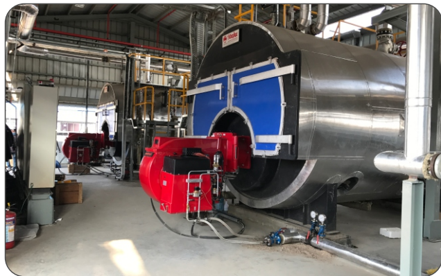
Daramic, LLC - Dahej, Gujarat Steam Boiler(IBR):- Capacity- 6 TPH x 2, Fuel- Furnace Oil cum Natural Gas
