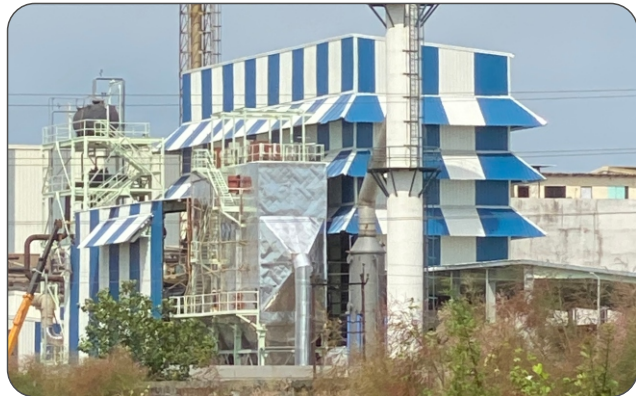
SML Ltd. - Surat, Gujarat Thermic Fluid Heater:- Capacity- 60,00,000 Kcal/hr, Fuel- Coal
