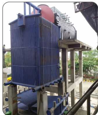
Benzo Chem Industries Pvt. Ltd. - Dahej, Gujarat Steam Boiler(IBR):- Capacity - 10 TPH, Fuel - Coal
