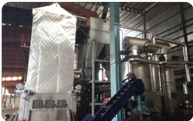
Chakradhar - Surat, Gujarat Steam Boiler(IBR):- Capacity - 8 TPH, Fuel- Coal
