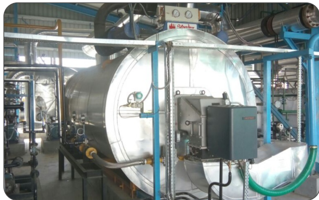
Bostik India Pvt. Ltd. - Bharuch, Gujarat Thermic Fluid Heater:- Capacity - 20,00,000 Kcal/hr, Fuel - Natural Gas
