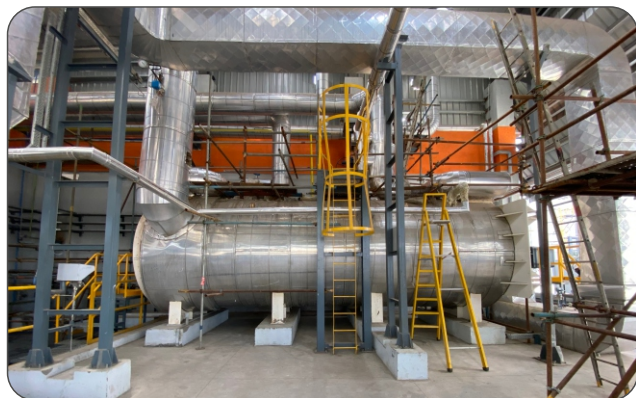
Aarti Industries - Dahej, Gujarat Thermic Fluid Heater:- Capacity- 40,00,000 Kcal/hr x 2, Fuel- Natural Gas
