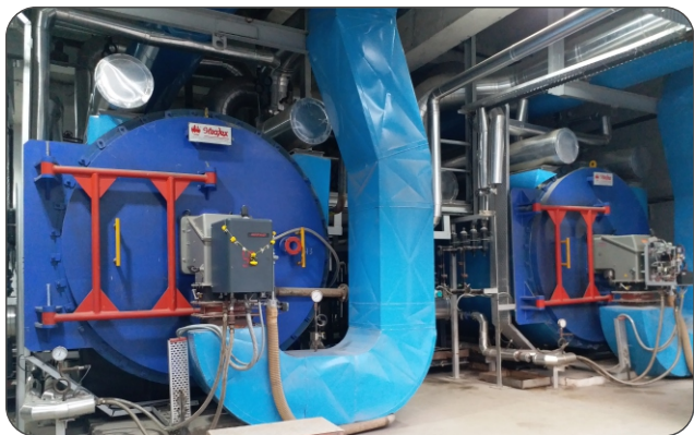
SML Ltd. - Surat, Gujarat Thermic Fluid Heater:- Capacity- 25,00,000 Kcal/hr x 2, Fuel- Furnace Oil cum Natural Gas
