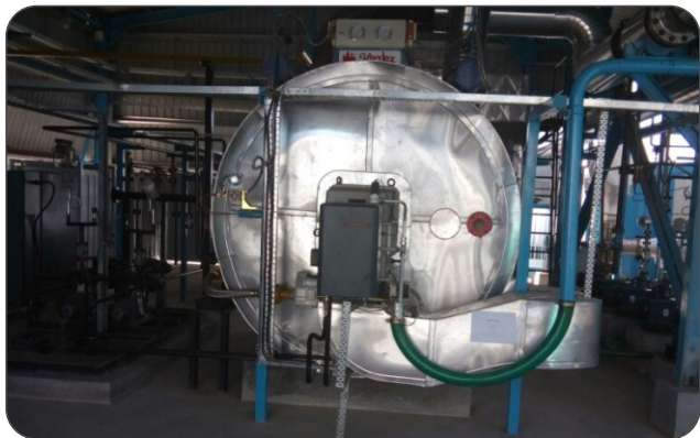
Bostik India Pvt. Ltd. - Bharuch, Gujarat Thermic Fluid Heater:- Capacity - 20,00,000 Kcal/hr, Fuel - Natural Gas
