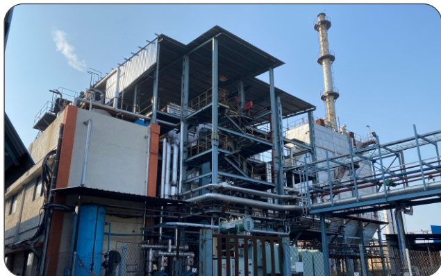
Camlin Life Science - Dahej, Gujarat Steam Boiler(IBR):- Capacity - 20 TPH, Fuel - Coal / FBC
