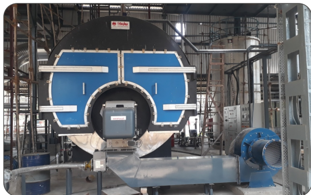
Amines & Plasticizers Ltd. - Mumbai, Maharashtra Steam Boiler(IBR):- Capacity- 12 TPH, Fuel- Natural Gas
