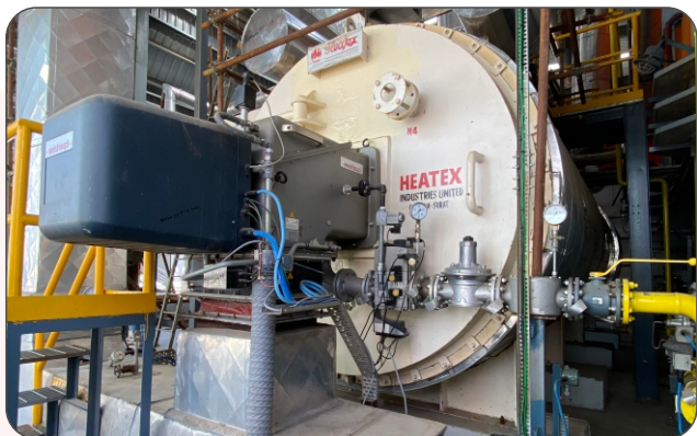
Aarti Industries - Dahej, Gujarat Thermic Fluid Heater:- Capacity- 40,00,000 Kcal/hr x 2, Fuel- Natural Gas
