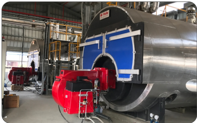
Daramic, LLC - Dahej, Gujarat Steam Boiler(IBR):- Capacity- 6 TPH x 2, Fuel- Furnace Oil cum Natural Gas
