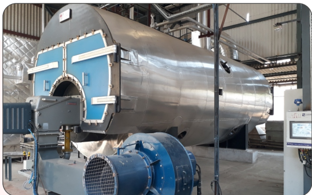
Amines & Plasticizers Ltd. - Mumbai, Maharashtra Steam Boiler(IBR):- Capacity- 12 TPH, Fuel- Natural Gas
