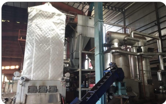
Chakradhar - Surat, Gujarat Thermic Fluid Heater:- Capacity- 20,00,000 Kcal/hr, Fuel- Coal
