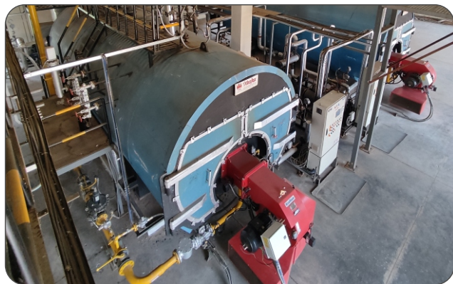
NDDB - Odisha Steam Boiler(IBR):- Capacity - 8 TPH x 2, Fuel- LPG / LDO
