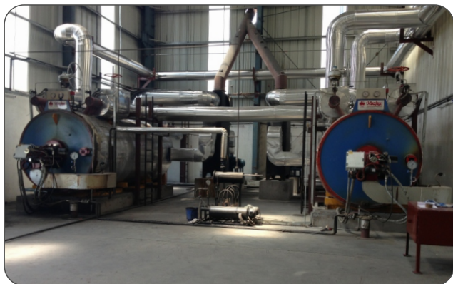
Tapadia - Nagpur, Maharashtra Thermic Fluid Heater:- Capacity- 15,00,000 Kcal/hr, Fuel- Coal
