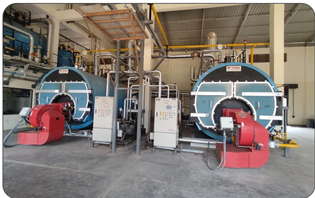
NDDB - Odisha Steam Boiler(IBR):- Capacity - 8 TPH x 2, Fuel- LPG / LDO
