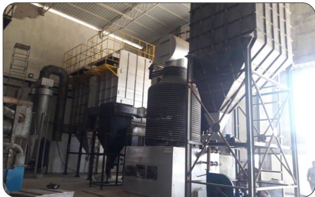
Ovel Laminates Pvt. Ltd. - Rajkot, Gujarat Thermic Fluid Heater:- Capacity- 15,00,000 Kcal/hr, Fuel- Coal
