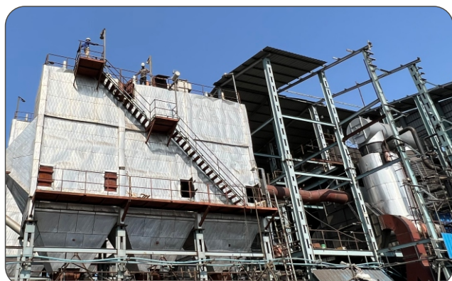
Camlin Life Science - Dahej, Gujarat Thermic Fluid Heater:- Capacity- 50,00,000 Kcal/hr, Fuel- Coal
